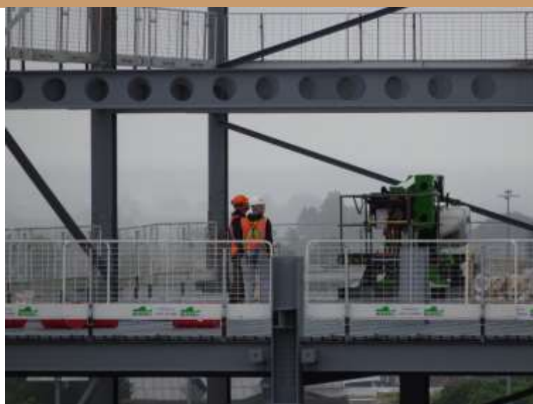
📍 Council offices at Friargate under construction
